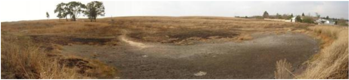
Photograph 3: Artificial Dam on the southern section of the proposed site.
