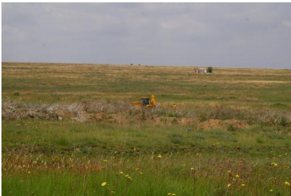
Photograph 7: Construction activities that took place within the wetland area.
