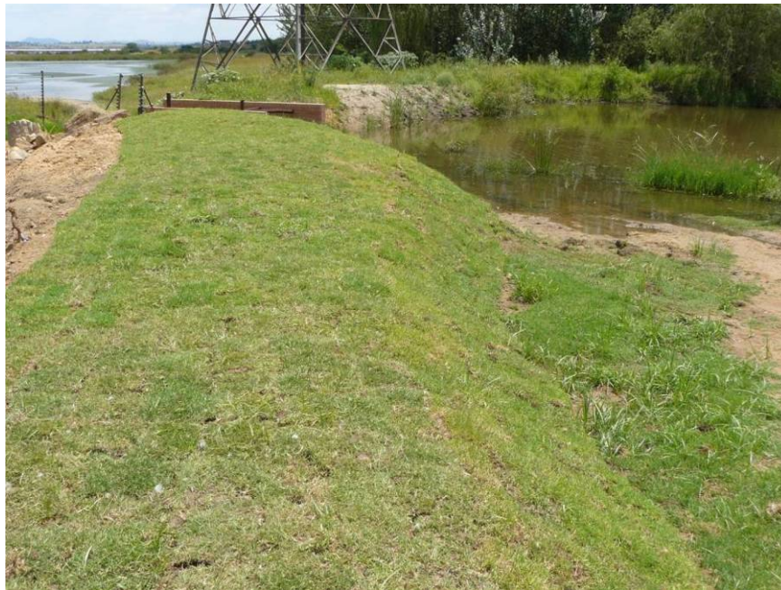
Figure 3: A recently-made weir in the drainage line with newly-planted Kikuyu grass.
